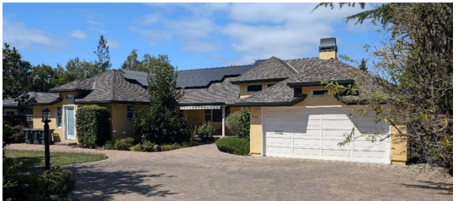
Figure 10: The all-electric retrofitted home.
